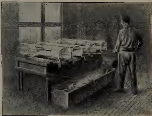
FIG. 152. Third step in making window glass: cutting the cylinders
